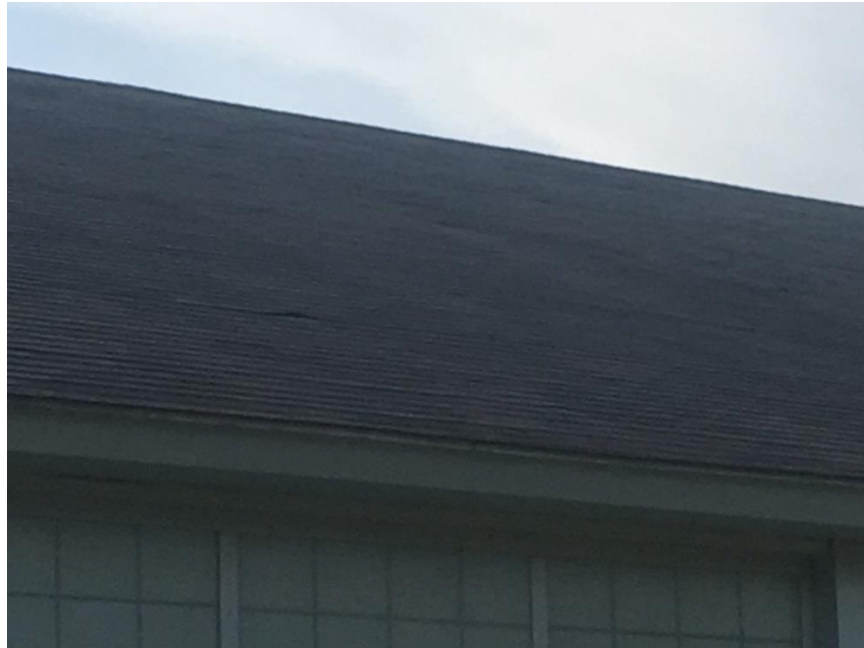
Barnstable West Barnstable Roof
