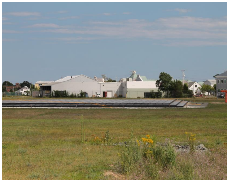
Engineered Material Arresting System (EMAS) or Runway SAFE System
