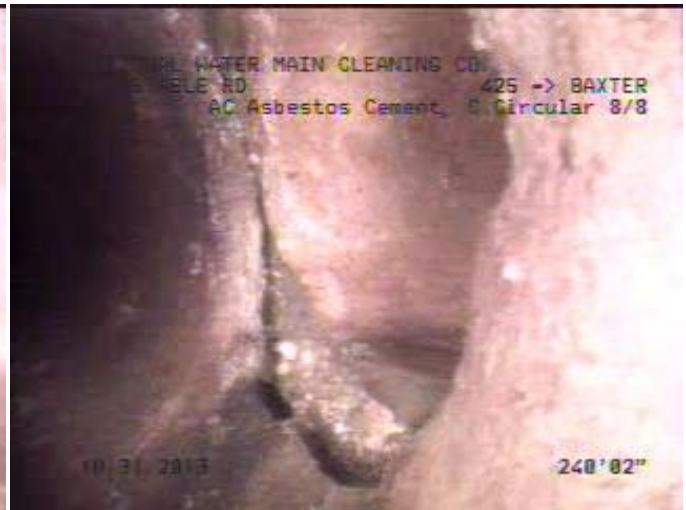
Internal View of Pipe Corrosion
