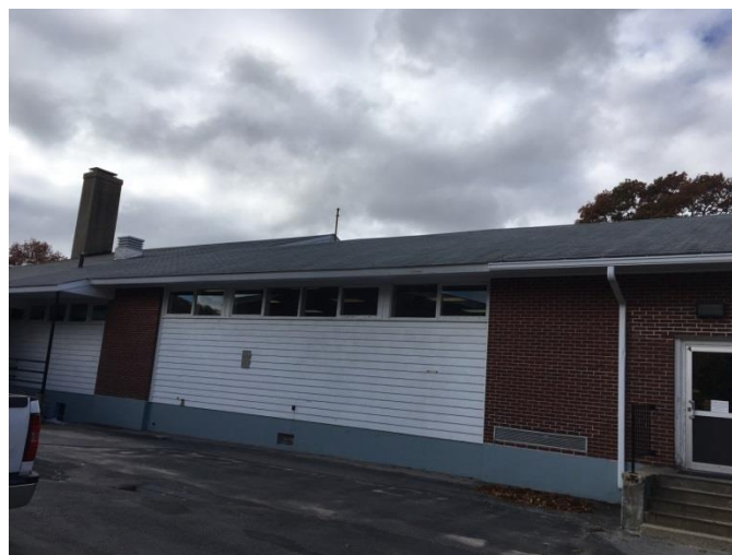
Centerville Elementary Roof Replacement
