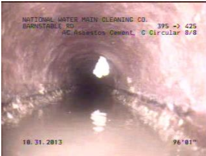
Internal View of Pipe Corrosion
