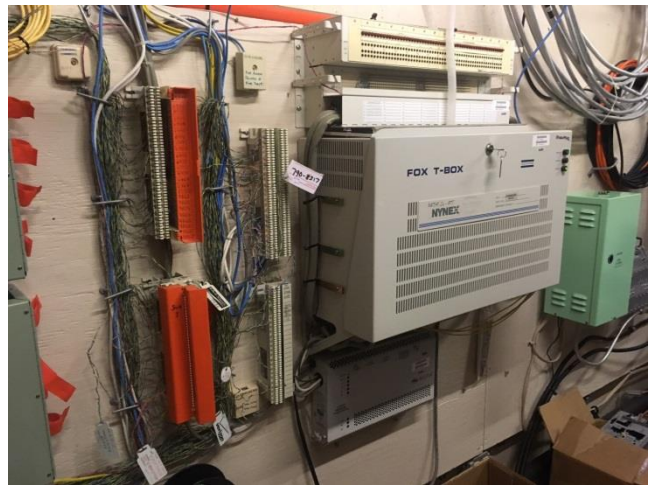
Typical DVR/Camera Security System and Current Barnstable High School Phone Switch
