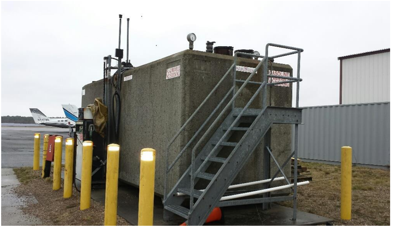
Existing Con-Vault and Gas Boy
