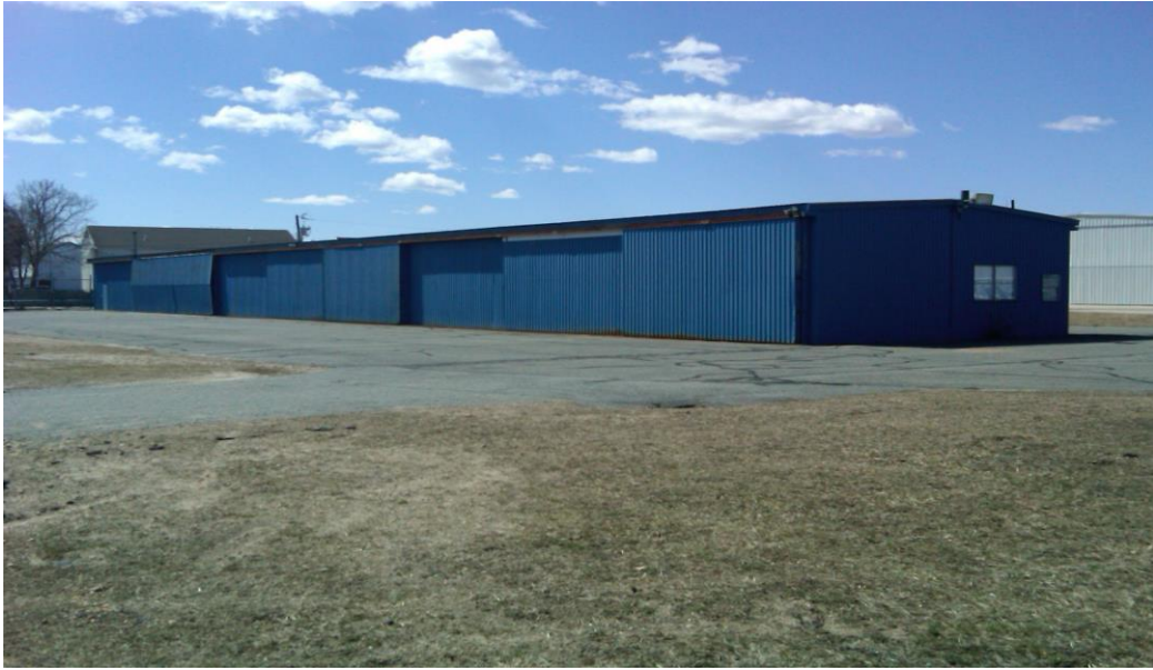
Recently demolished T-Hangar
