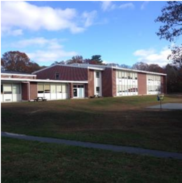
Centerville Elementary School Windows
