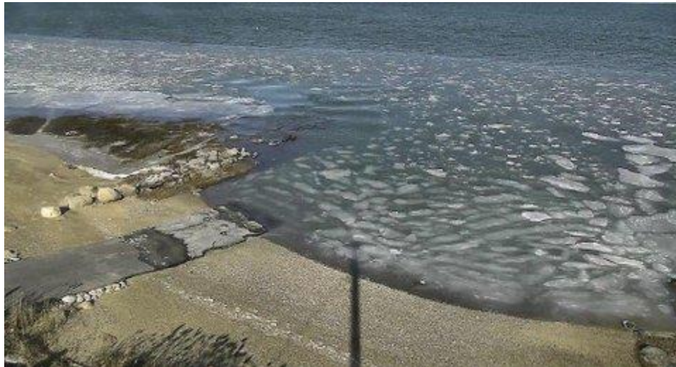
Scudder's Lane Boat Ramp
