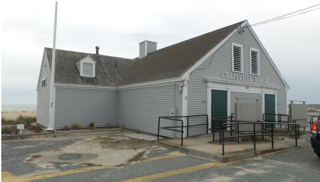
Craigville Bathhouse: Location of New Waste Water Pump Station On Side of Building
