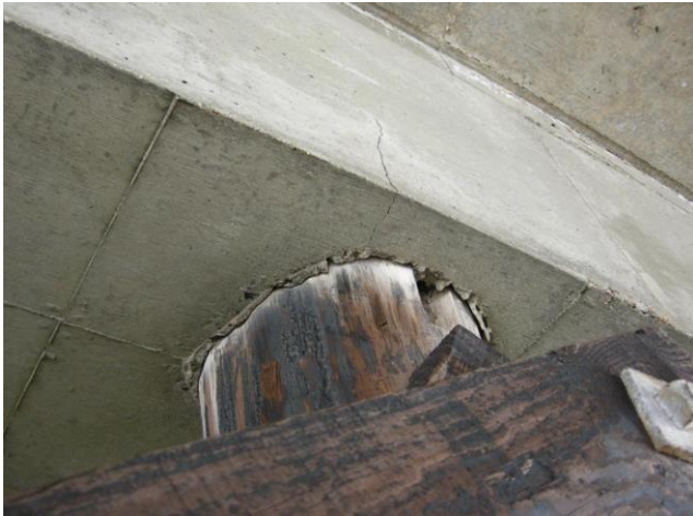
Bumps River Bridge Support Beams
