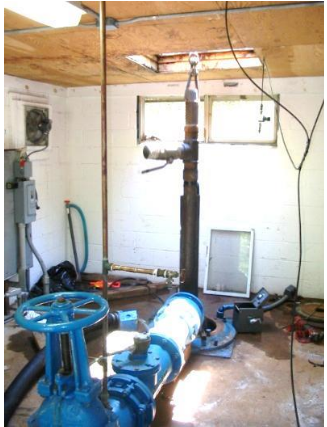
Upgrade Pump Stations
