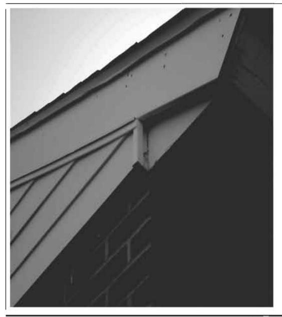
TYPICAL EXIST GABLE END WITH VINYL SIDING & TRIM, NEW RAKE BOARD, & METAL DRIP FLASHING.
