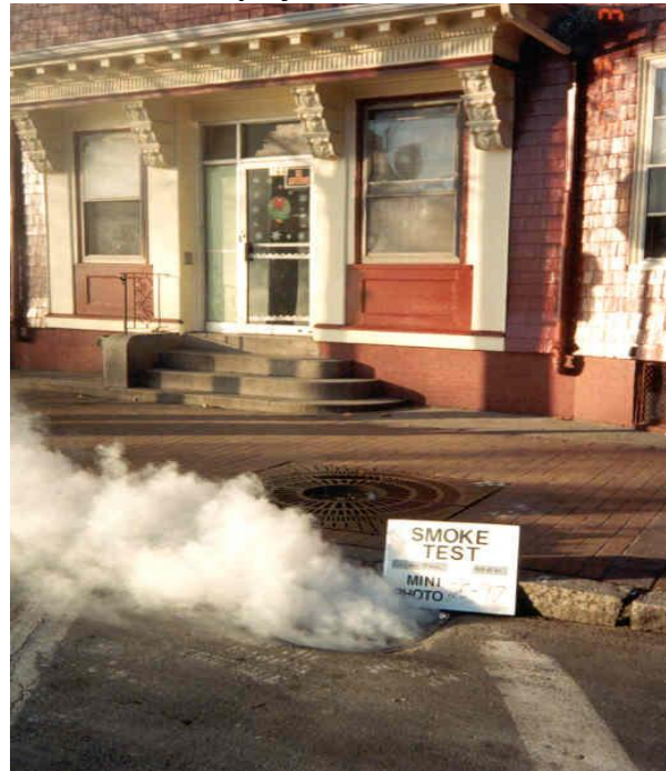
Catch basin tied directly into sanitary sewer system.
