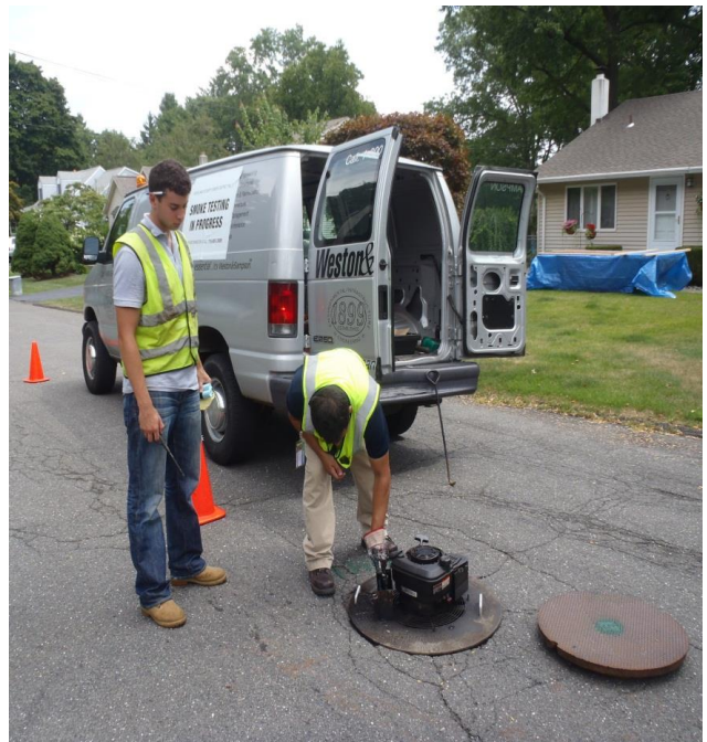
Setup of smoke blower.
