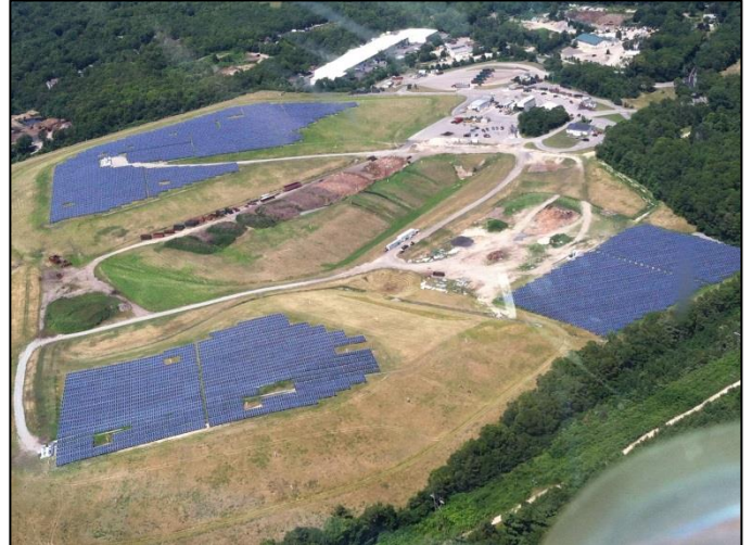
Solid Waste Facility – Aerial View
