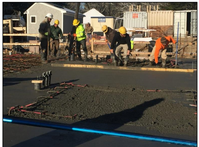
Maher Filtration Under Construction
