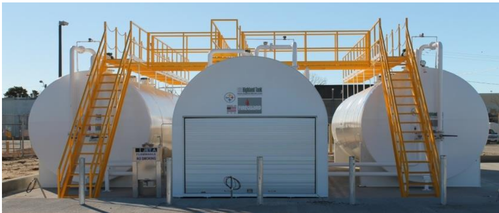
New Airport Jet Fuel Storage Facility 2016
