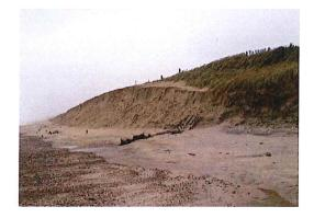
This picture is from November  $2^{nd}$  looking east You can see at the tow of the dune shows the conduit. The material in front – up to the grass – is the "sacrificial sand." There is about 1/3 of the sand left from what was placed there last year.
