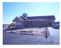
This is the front view of the bathhouse. The siding is up and the roof shingling is complete. The cupola is up. Brass on top of cupola is there.
