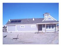
This picture shows the back of the bathhouse. The overhang gives the appearance that the building is bigger but it is the same footprint. The solar panels are for hot water showers.
