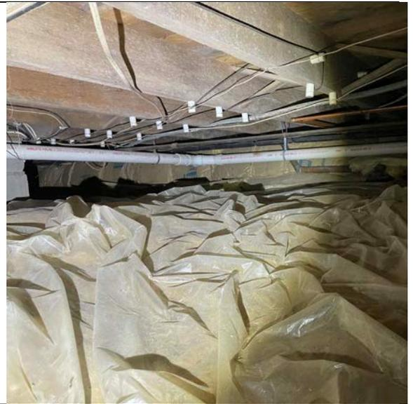
P6: Repaired First floor framing with temporary Posts
