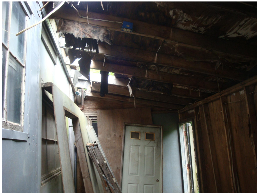
View of Section at the Rear of the Building in Poor Condition
