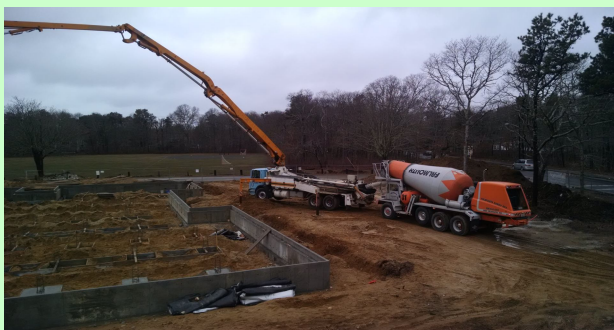
Building foundations are poured at CELC jobsite
