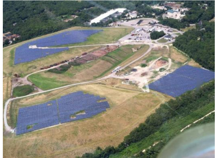
Solid Waste Facility – Arial View
