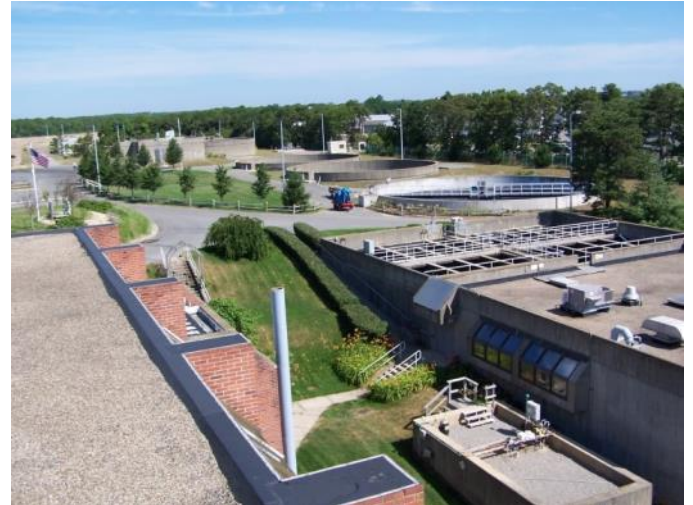
Water Pollution Control Facility – Buildings
