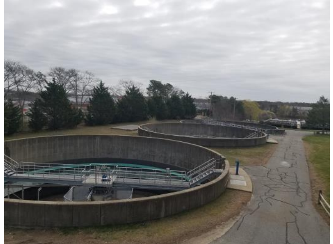
Water Pollution Control Facility – Secondary Clarifiers
