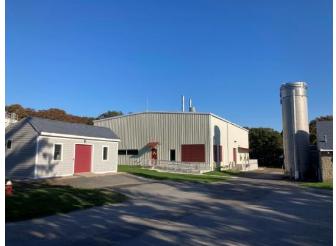
Harold E. Tobey Maher Water Filtration Plant
