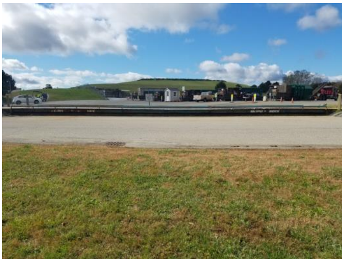
Solid Waste Facility
