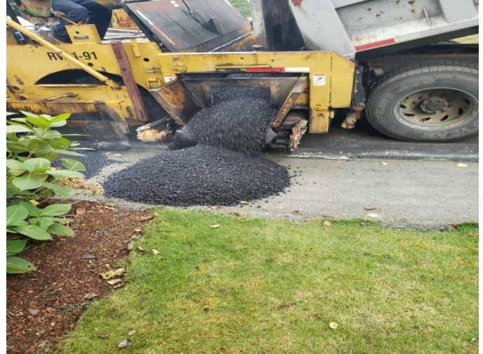
Glen Eagle Drive Road Project
