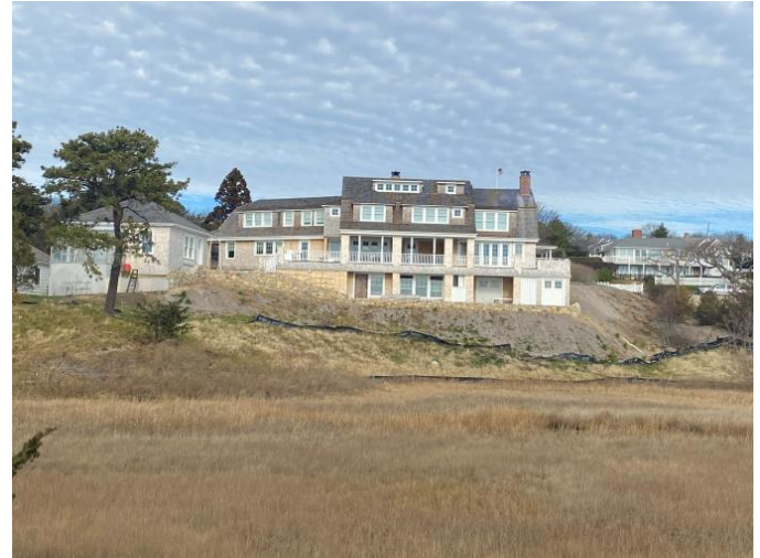
Atlantic Avenue Renovation
