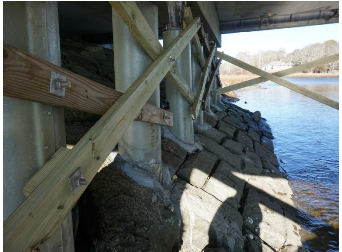
Bumps River Bridge Construction
